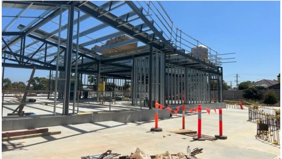
Steel works for the new pavilion and tennis and bowling club
