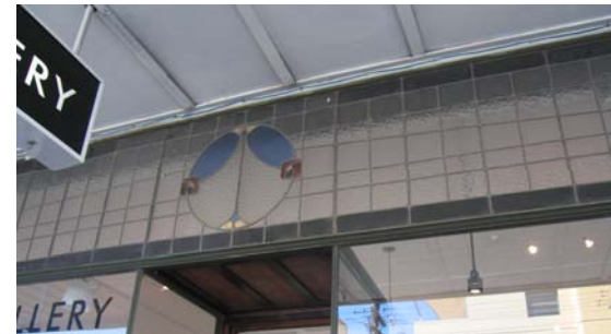
Leadlight detail of Interwar shopfront
