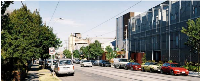
Existing streetscape along Waverley Road within the DDO5 area
