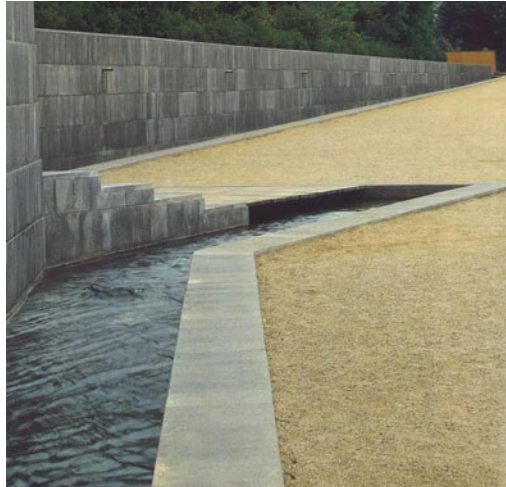
Epoxy bonded gravel
