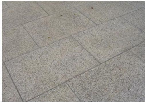
Precast unit pavers with sandblasted finish in stretcher bond pattern as used in New Quay East (uniform colour)
