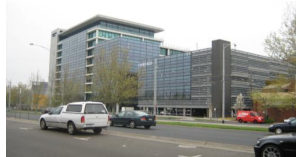
Figure 4.1: View south-east across Dandenong Road towards Monash University building
