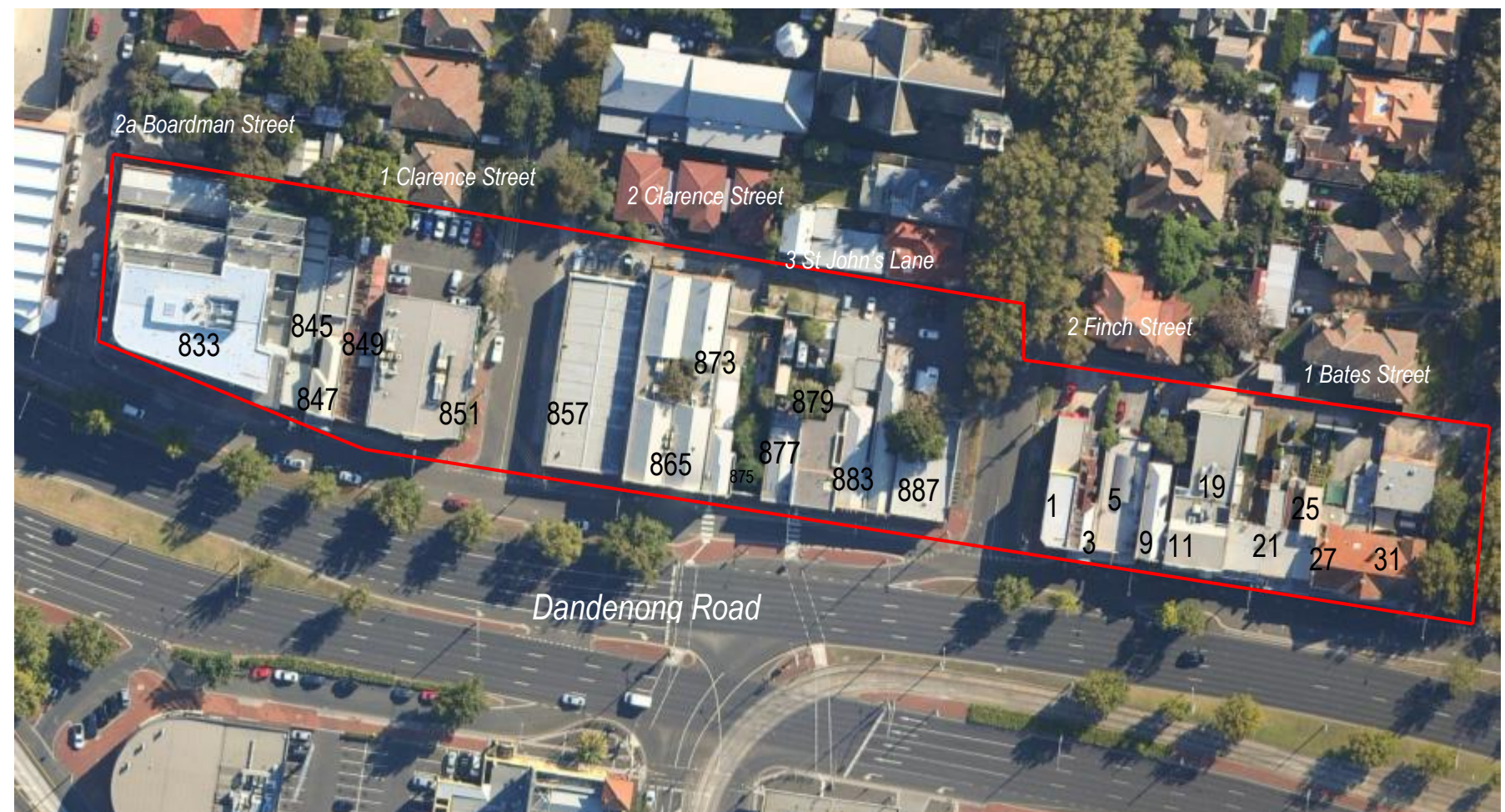
Figure 3.7: Aerial Photo of Precinct B
