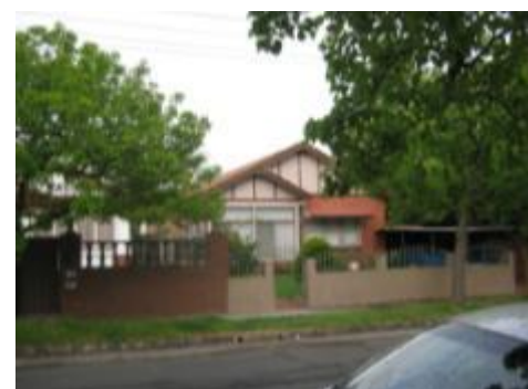
Figure 3.3: Dwelling on south side of John Street
