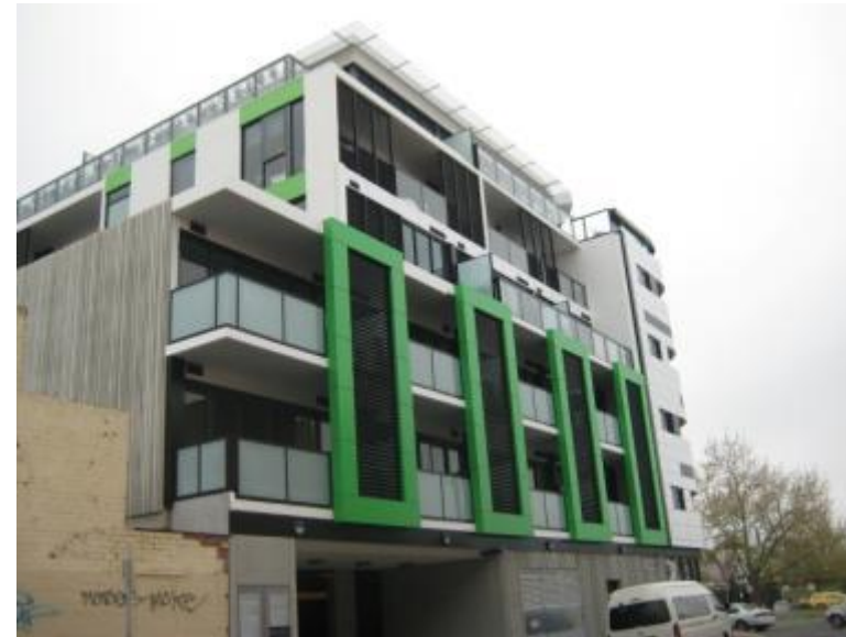
Figure 3.5: Recent 6 storey development at 833-843 Dandenong Road
