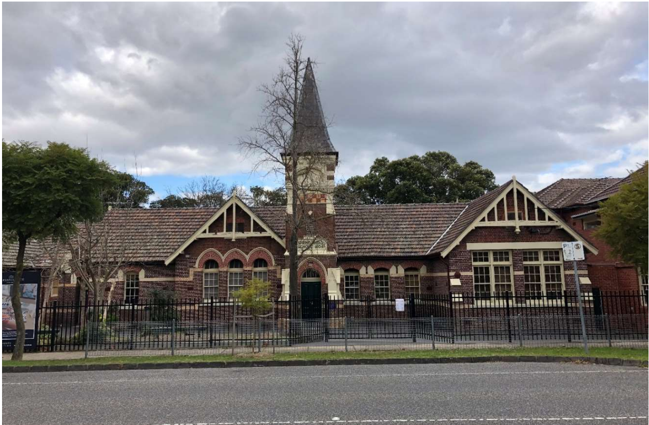
Figure 1. Primary School No 1604 – 2B Spring Road, Malvern (GJM Heritage, July 2020).
