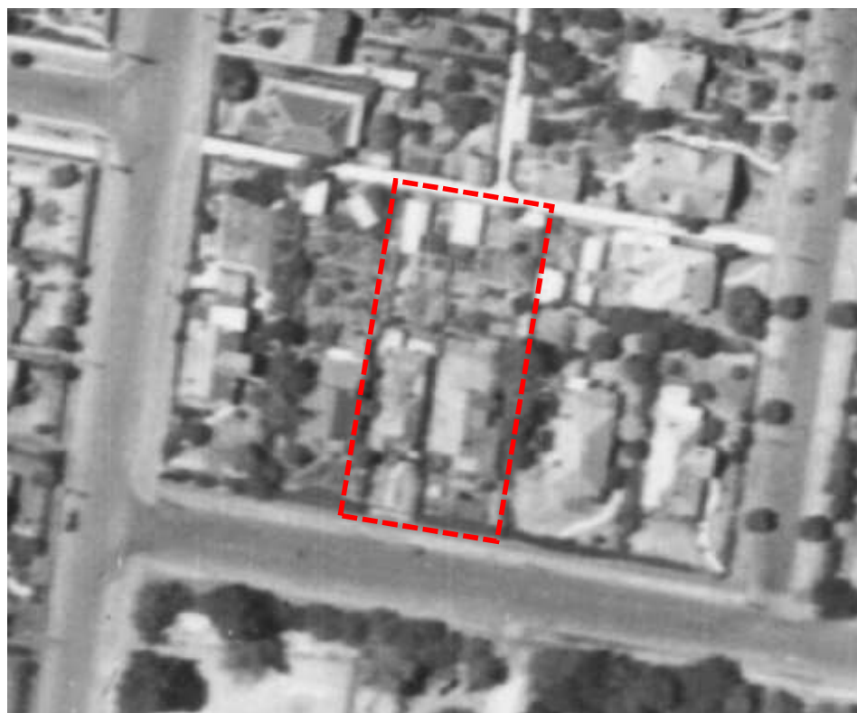
Figure 5. Aerial photograph showing 5 and 7 Ascot Street, 1945 prior to the construction of the existing flats, indicated by red outline (Landata)
