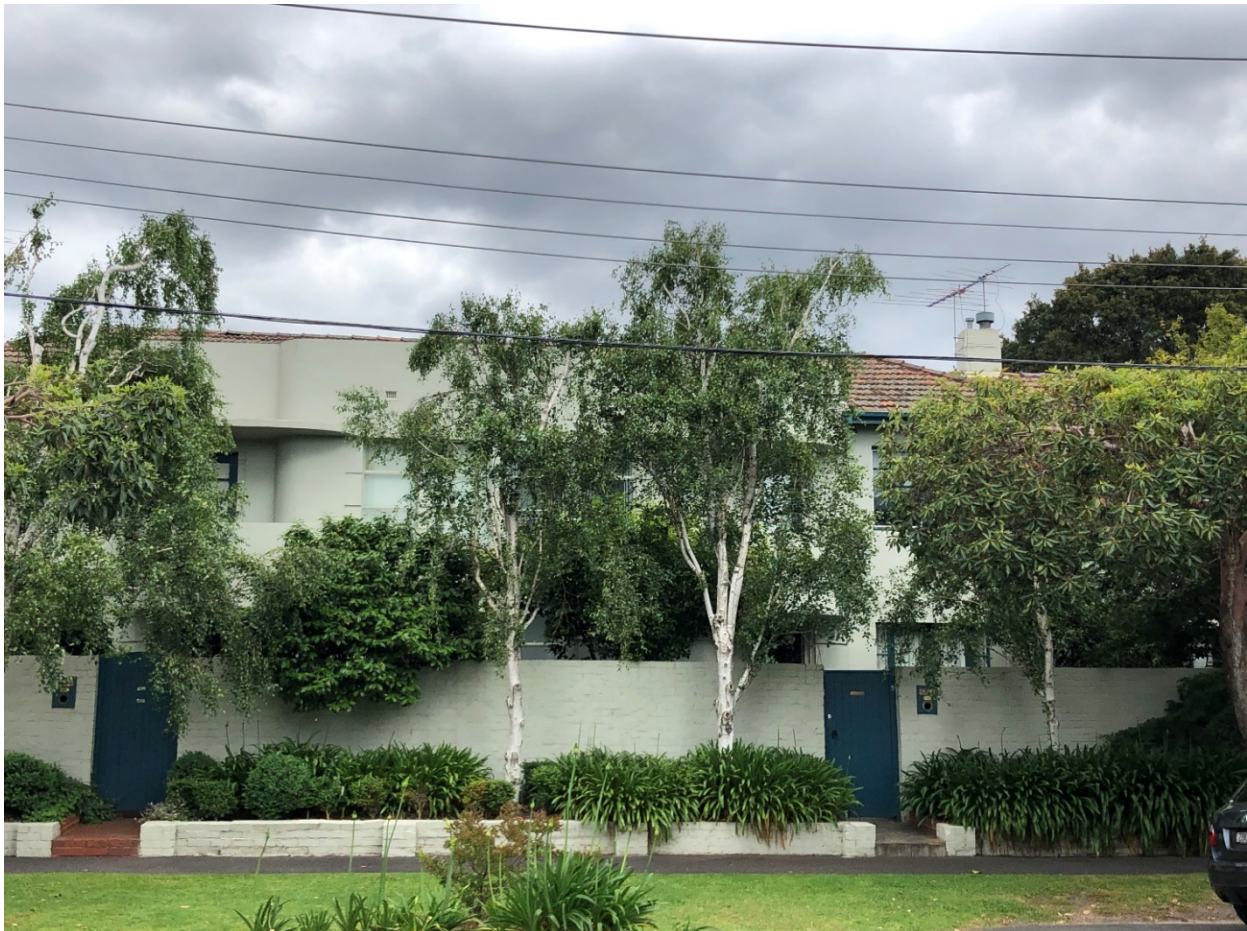
Figure 1. 79 Stanhope Street (eastern elevation), Malvern (December 2020)
