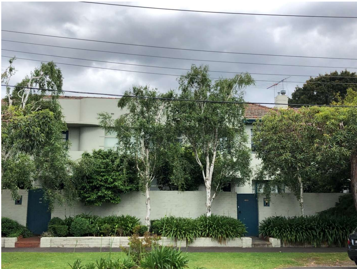
Figure 1. 79 Stanhope Street, Malvern (eastern elevation) (GJM Heritage, December 2020).
