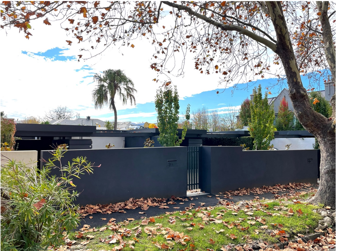
Figure 1. 11-13 Sorrett Avenue, Malvern (May 2021)
