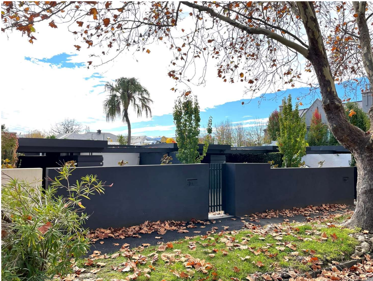
Figure 1. 11-13 Sorrett Avenue, Malvern (GJM Heritage, May 2021).
