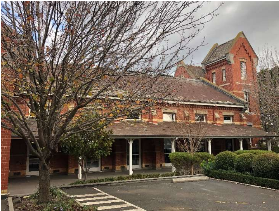
Figure 4. North elevation of hall (Source: GJM Heritage, July 2020)
