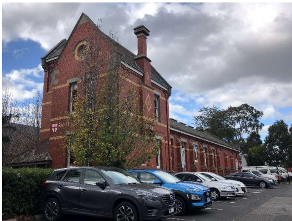
Figure 3. Parish Hall (GJM Heritage, July 2020).
