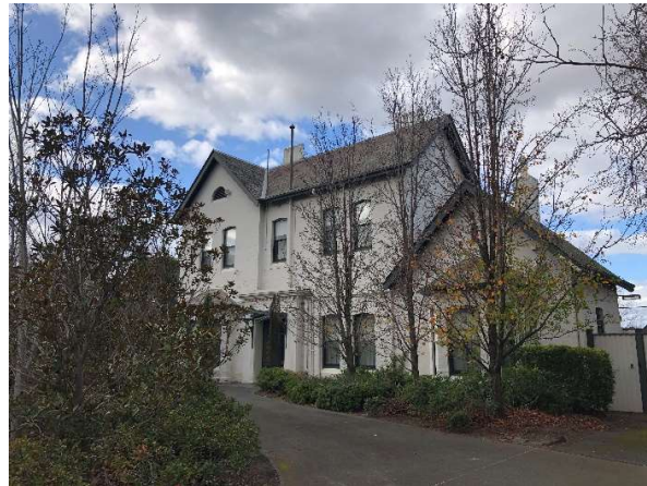
Figure 2. Vicarage (GJM Heritage, July 2020).
