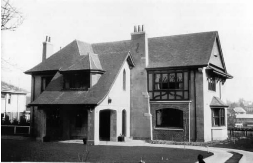
Figure 4. House soon after completion, c1928. (Source: SHC MP746).
