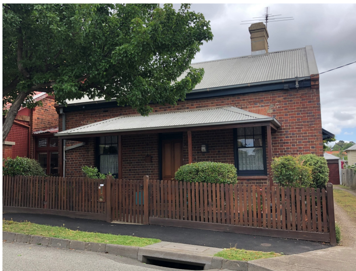
Figures 1 & 2. 1 Cawkwell Street (top), and 3 Cawkwell Street (bottom) Malvern (GJM Heritage, July & November 2020).
