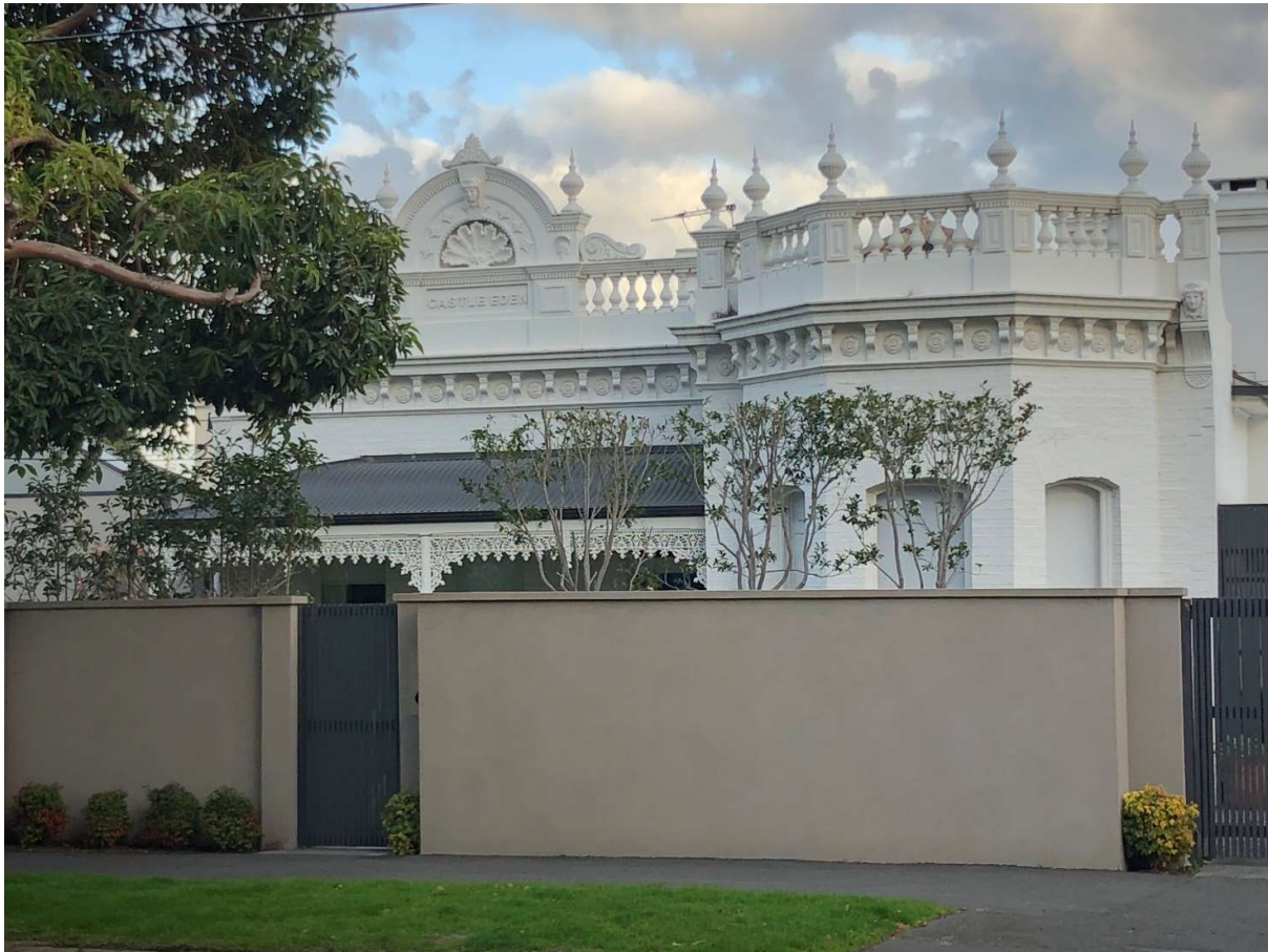
Figure 1. 54 Stanhope Street, Malvern (GJM Heritage, July 2020).
