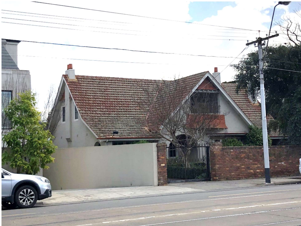
Figure 1. 333 Glenferrie Road, Malvern (GJM Heritage, July 2020).
