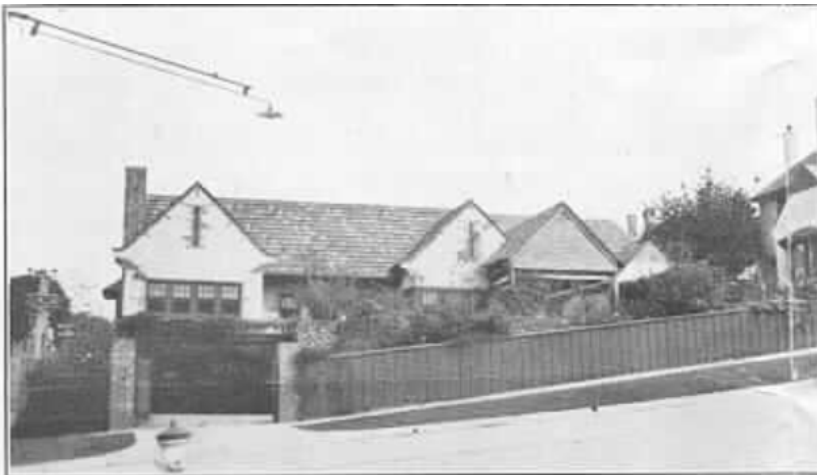
Figure 4. House at 1 Henderson Avenue, photo dated c1935 (SHC, MP5288).
