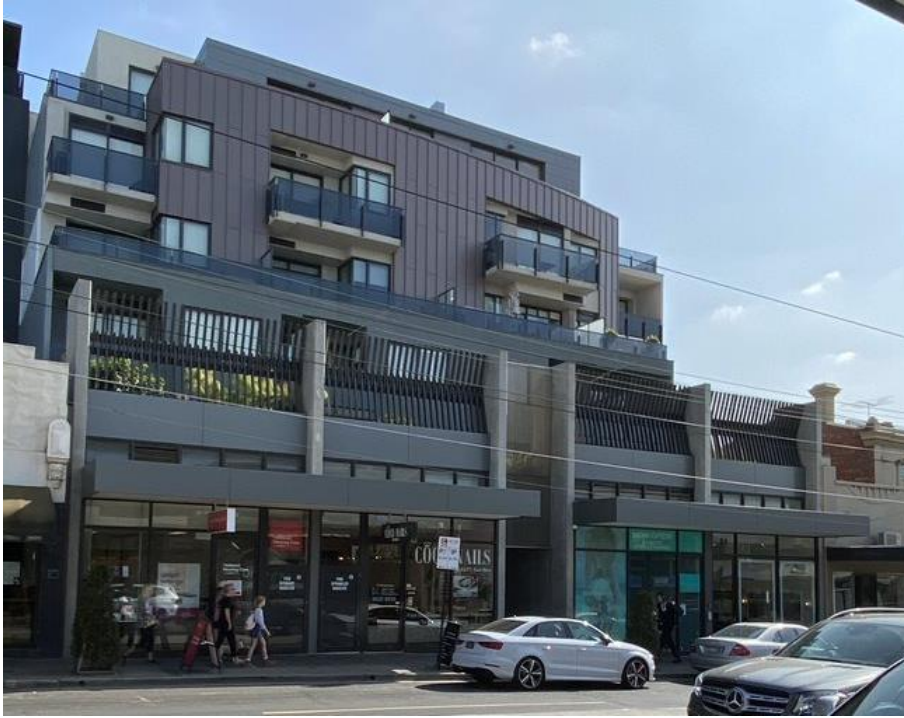
Figure 19. Contemporary infill development set back from the Toorak Road (north side) street frontage between Caroline Street to Avoca Street. (Source: Context, February 2020)
