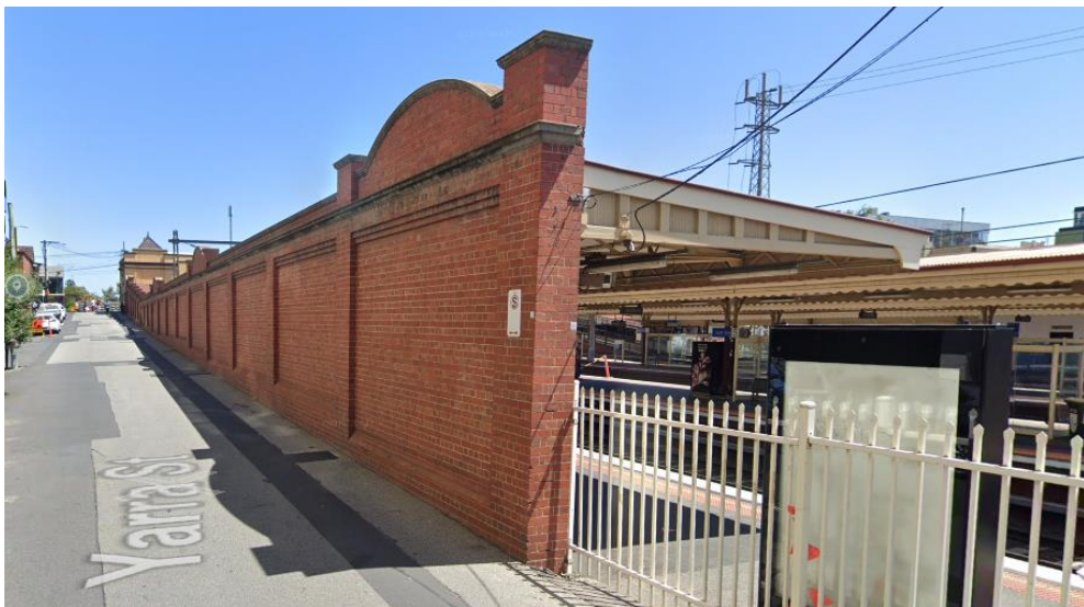
Figure 27. Red face brick wall on the western side of Yarra Street supporting the canopy on platform 6 (Source: Google January 2019)
