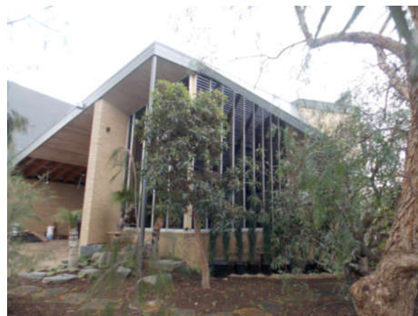
Figure 10: Recent view of the street frontage, showing full-height window wall to lobby/stairwell Source: photograph by Built Heritage Pty Ltd
