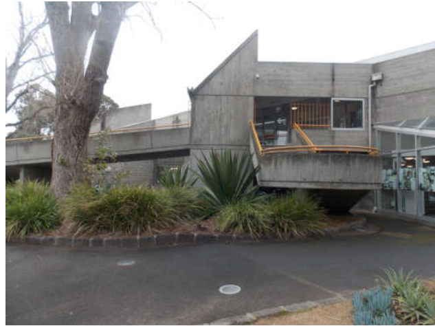
Figure 14: Harold Hold Memorial Swimming Pool, by Kevin Borland & Daryl Jackson in association (1966-69) Source: photograph by Built Heritage Pty Ltd
