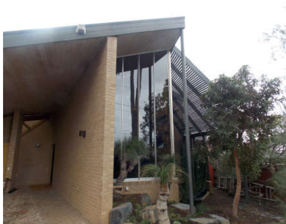
Figure 9: Recent view of the street frontage, showing the bold skillion roof to the carport side Source: photograph by Built Heritage Pty Ltd
