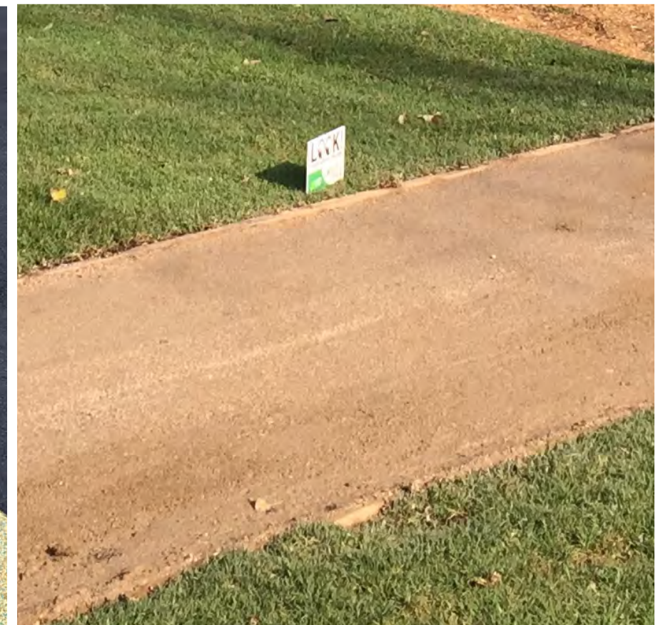
Compacted granitic gravel path
