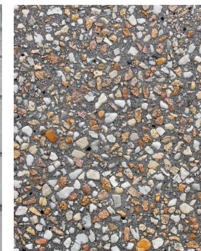
Exposed aggregate pavement
