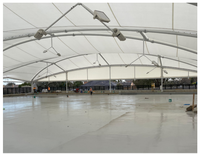
View of the bowling green with canopy and lighting installed
