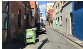
Narrow pathways blocked by bins from commercial tenancies
