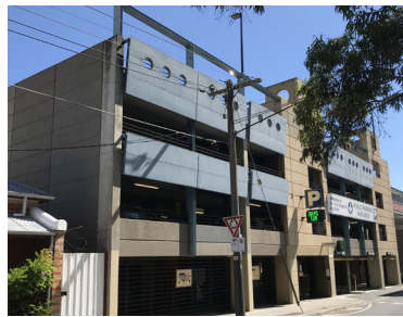
Council's Multi-level Carpark with pedestrian links to Cecil Lane and visual dominance of powerlines
