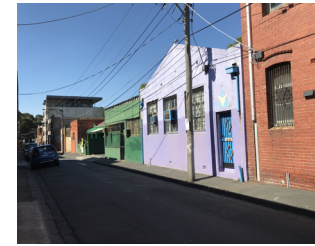
Overhead powerlines & wires
