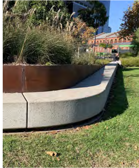
F02 - CONCRETE SEATING WALL, PRECAST EXPOSED AGGREGATE, 400mm HIGH, 500mm WIDE
