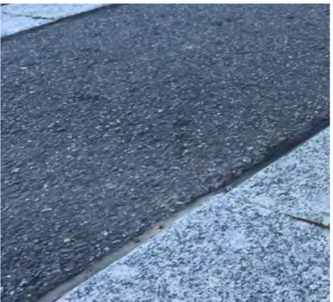
P04 - FEATURE STRIPE PAVER NATURAL STONE SILVER GREY GRANITE SIZE: 250X500x60mm GRADE: VEHICLE SOURCE: LOCAL GRANITE
