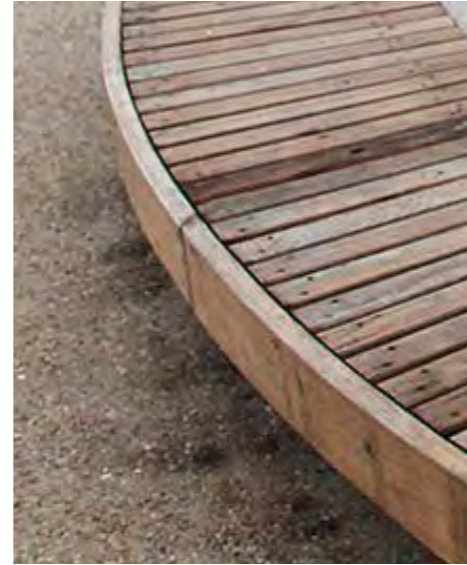
F03: CURVED BENCH 450mm HIGH, 600mm WIDE, SPOTTED GUM TIMBER ON STEEL FRAME
