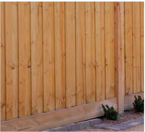
W02: STANDARD TIMBER FENCE EDGE TIMBER PALING FENCING 2500mm HIGH ALONG EDGES OF NEW POCKET PARKS.
