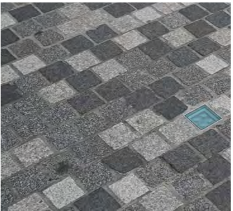
P03 - SHARED STREET PAVING NATURAL STONE 'SETT' PAVING IN TWO COLOURS, DARK GREY BLUESTONE AND SILVER GREY GRANITE SIZE: 100x100x90mm ARRANGED IN BOLD STRIPE PATTERN GRADE: VEHICLE SOURCE: LOCAL BLUESTONE AND GRANITE
