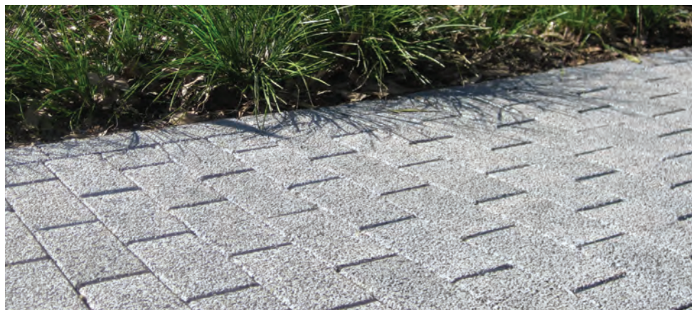
Bands of permeable paving used around raingardens
