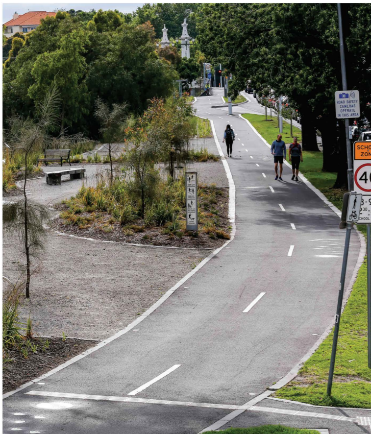
Shared Path - Asphalt with concrete edge
