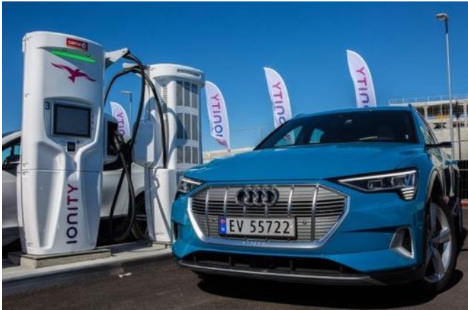
Figure 64 350kW ultra fast charger, Norway
