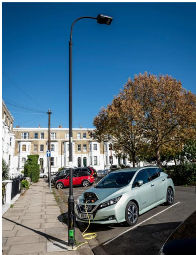
Figure 60 Lamp post charging, London
