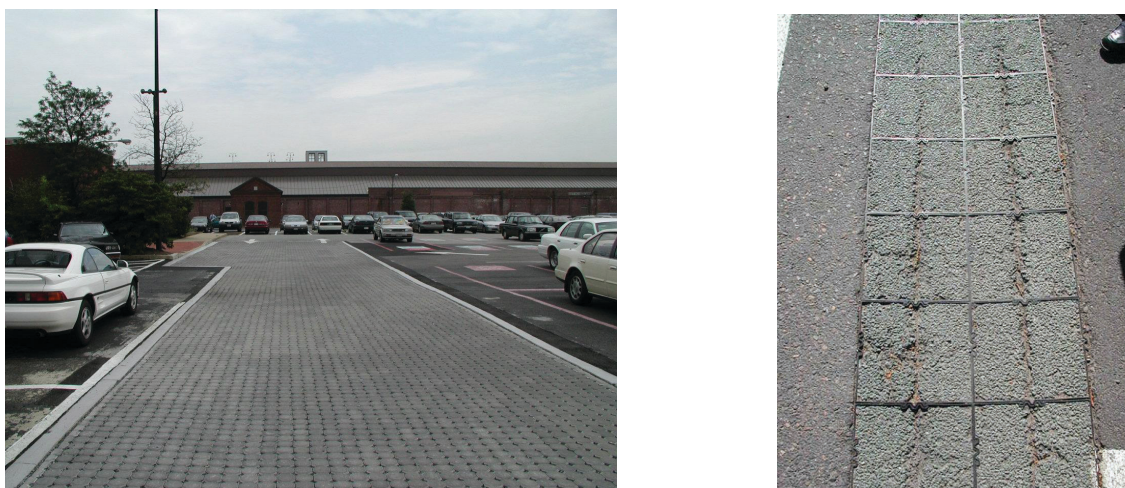
Figure 14.2 Examples of porous pavement: porous car park, Washington, DC, USA (Photo: Ecological Engineering); porous car park, road gutter, Manly, NSW (Photo: Tim Fletcher).
