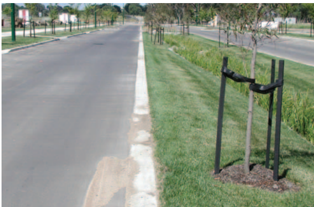
Figure 8.11 A flush kerb without setdown that shows accumulation of sediment on the street surface, and edge detail showing a recommended amount of setdown.
