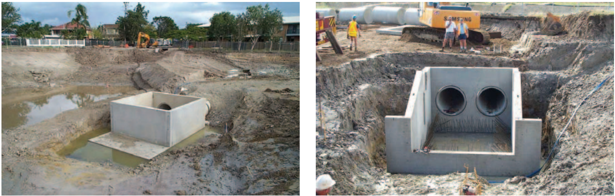
Figure 9.11 Connection inlet zone.
