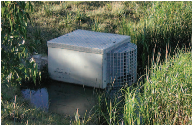
Figure 9.10 Debris guards on riser outlets.
