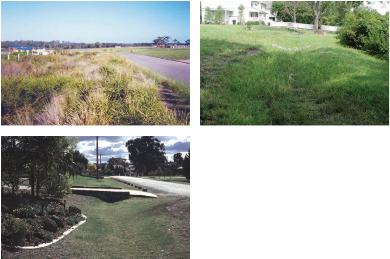
Figure 8.2 Swale systems: (L to R) heavily vegetated; use of check dams; grass swale with elevated crossings.
