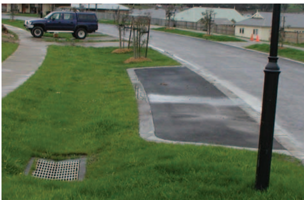
Figure 8.17 Similar buffer swale system for conveying runoff.
