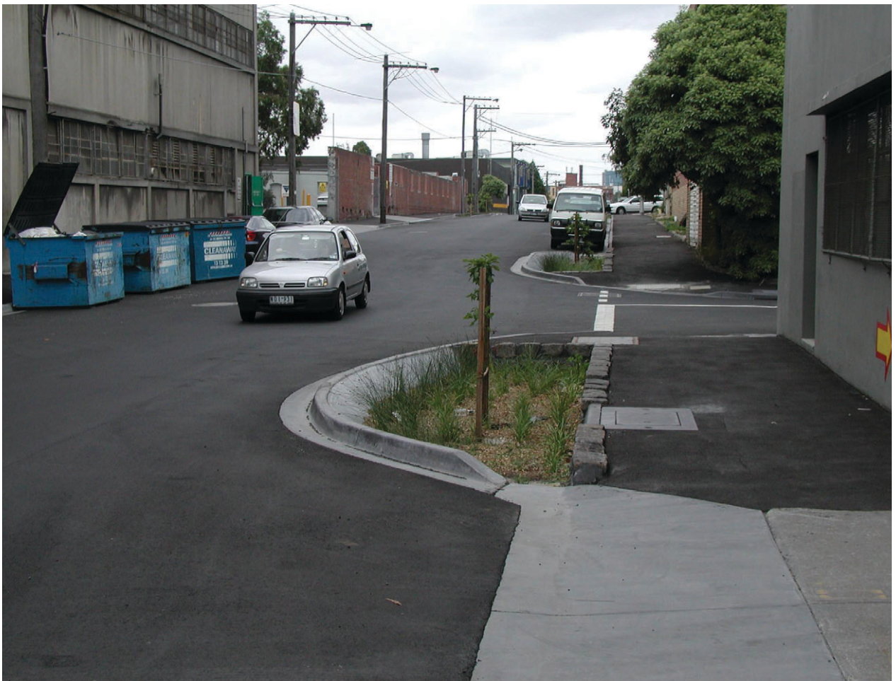
Figure 6.7 Retrofitted bioretention system in a street.
