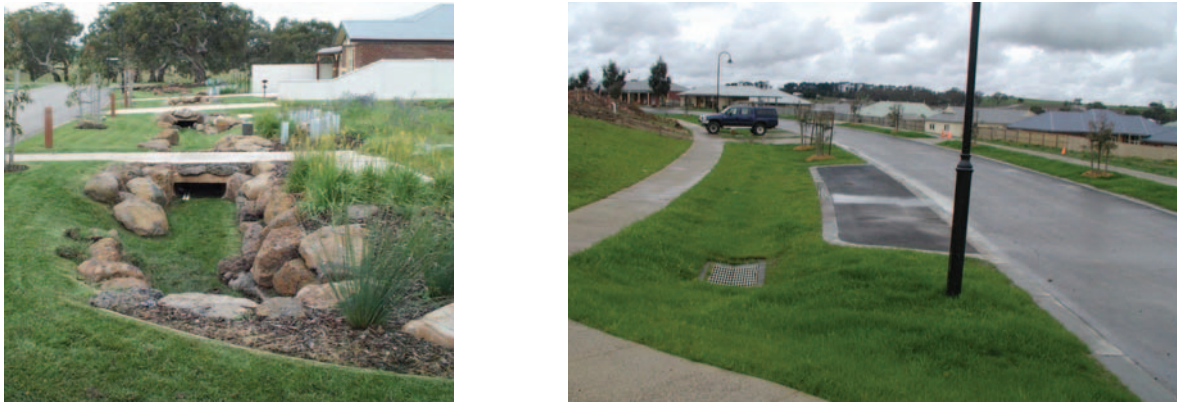
Figure 8.3 Elevated and at-grade driveway crossings across swales.
