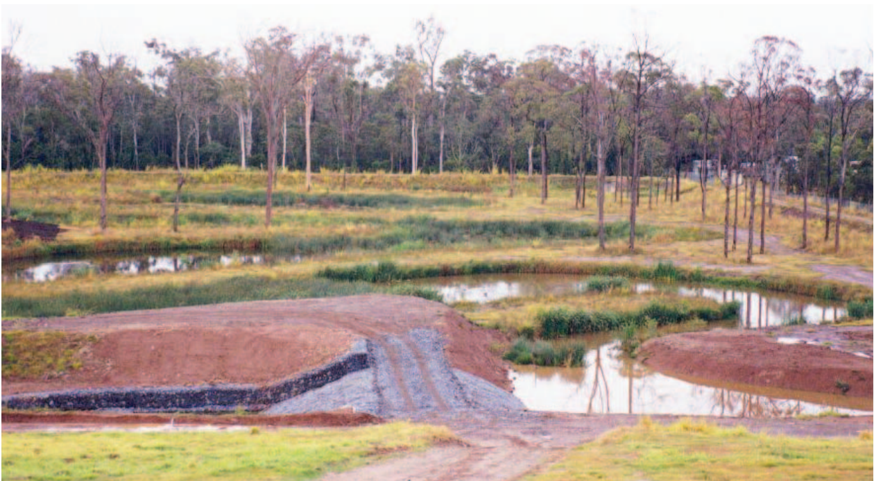
Figure 4.10 Overflow structure of a sedimentation basin.
