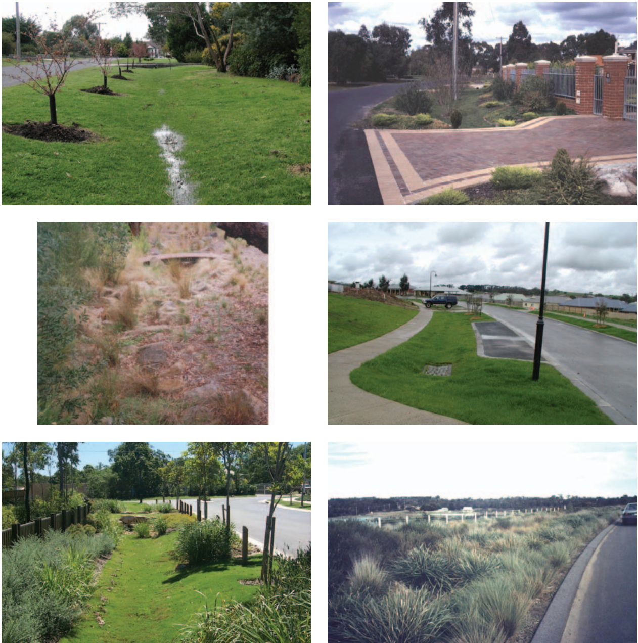
Figure 3.5 Swale vegetation is selected based on required appearance and treatment performance.
