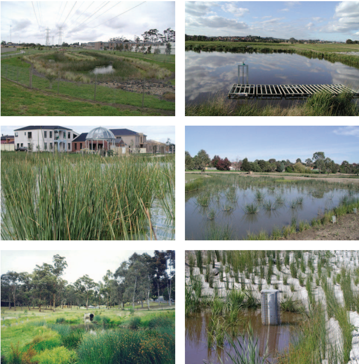
Figure 3.6 Wetlands can be constructed on many scales.
