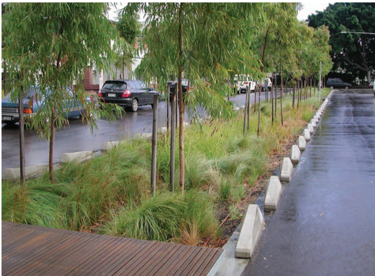
Bioretention swale in Zetland, NSW
