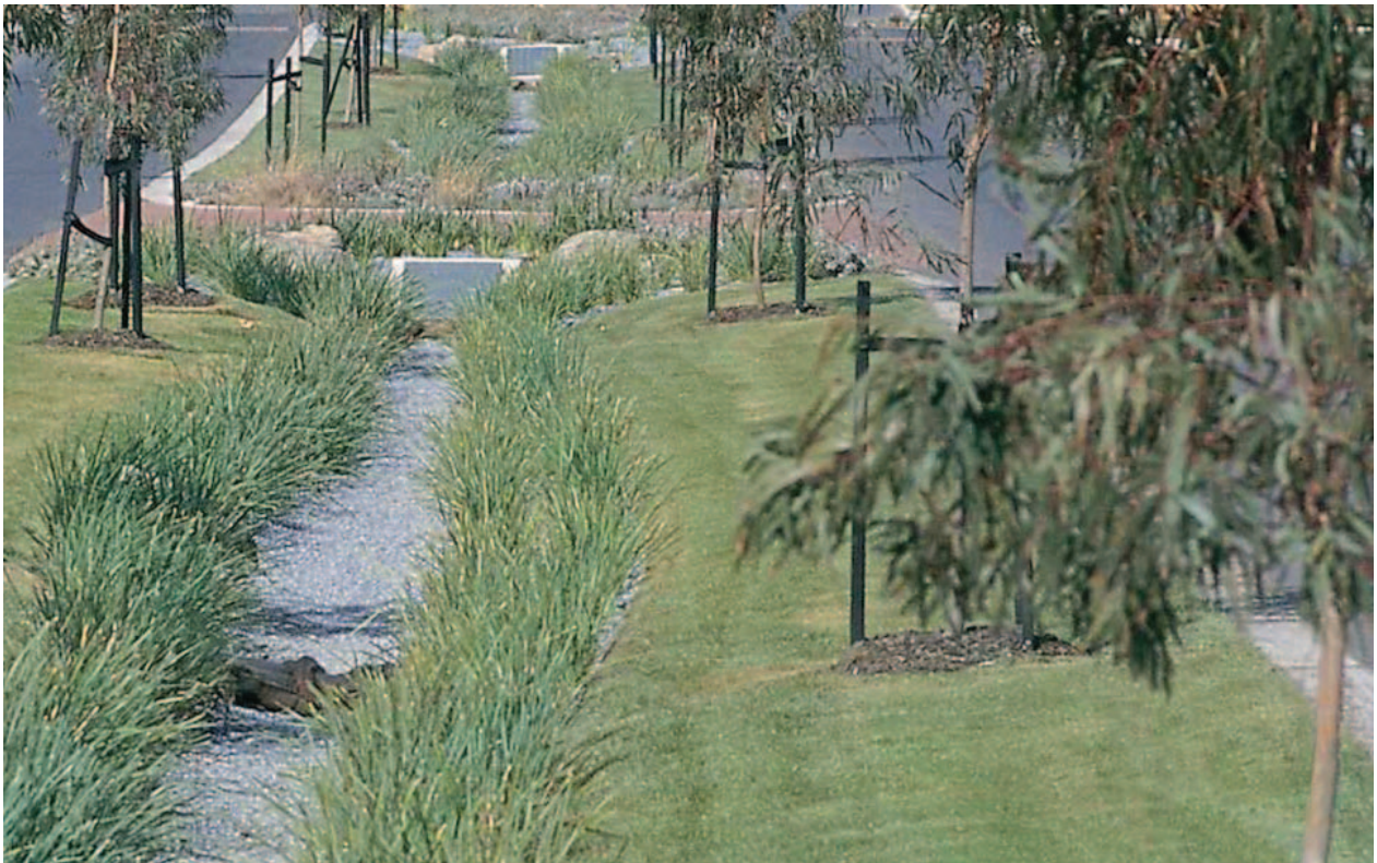
Figure 5.12 A bioretention swale.
