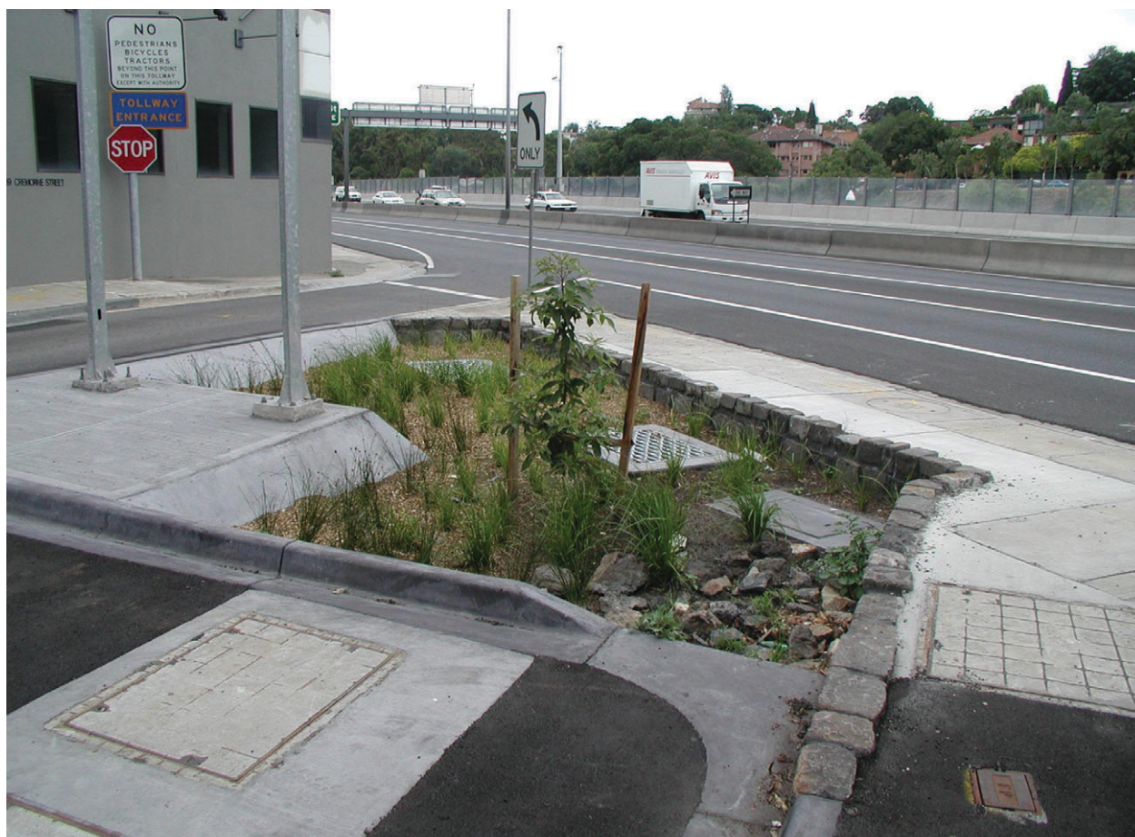
Bioretention basin in Richmond, Victoria.
