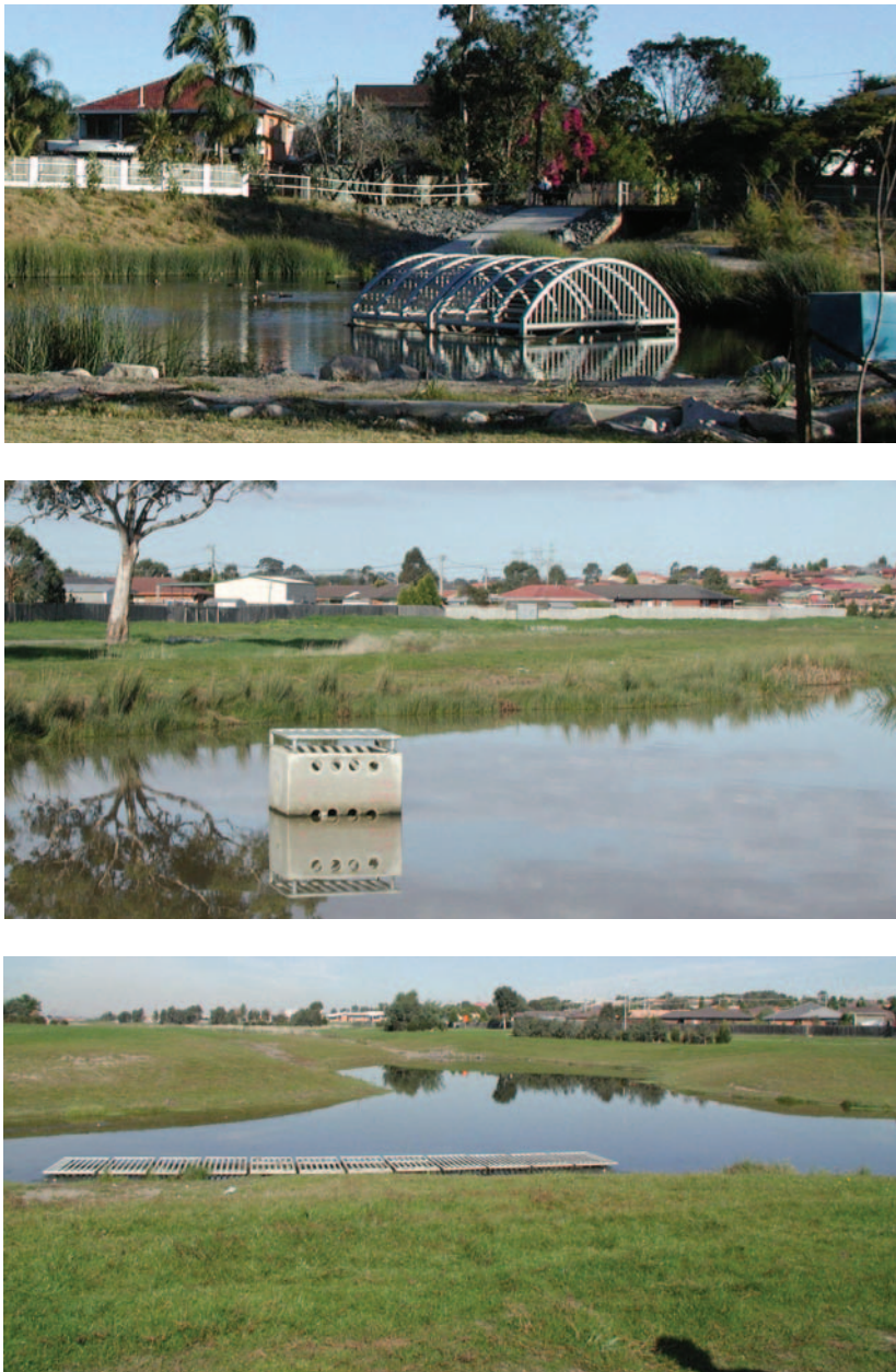
Figure 4.8 Debris protection for outlet pits.
