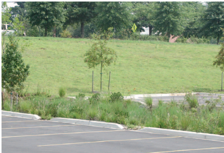
Figure 5.9 Kerbs with breaks to distribute inflows.
