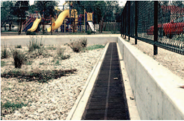
Figure 3.8 Infiltration systems are best suited to sandy soils with deep groundwater.
