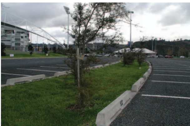
Figure 3.2 Bioretention swales are commonly located in median strips of roads and carparks
