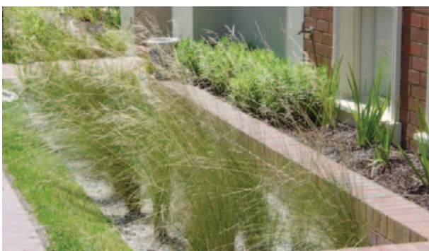
Figure 3.3 Bioretention basins are applicable at a range of scales and can be integrated with an urban landscape.
