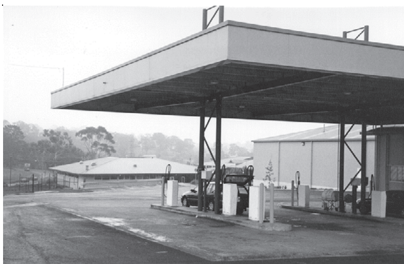
Figure 6.4 A fuelling area: paved, undercover area with a spoon drain to redirect surface run-off (City of Manningham).
