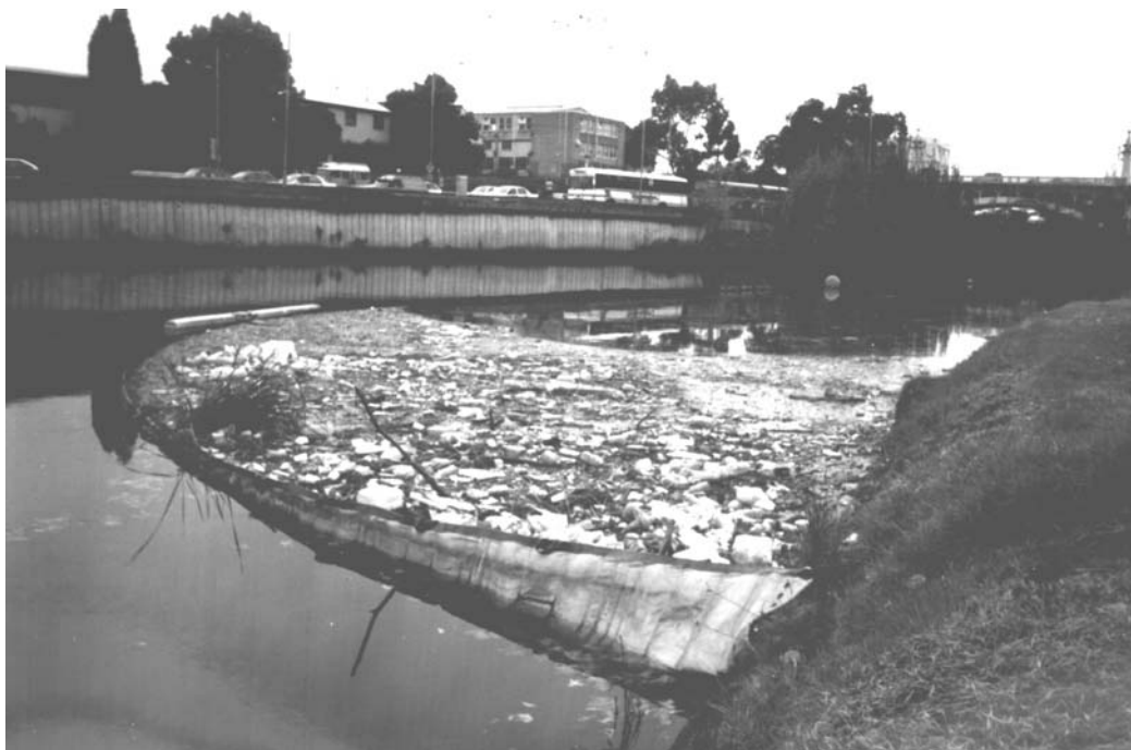
Figure 7.18 Flexible floating boom on the Yarra River, Melbourne.
