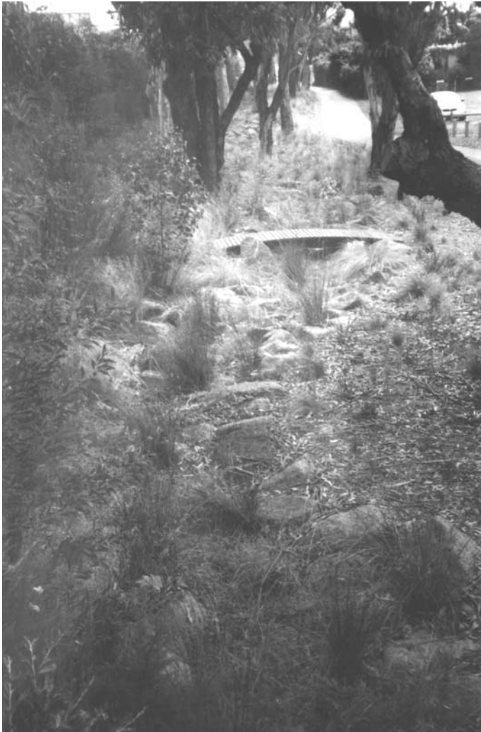
Figure 7.5 Swales (in this case, rock lined) promote infiltration, retard flows, improve water quality and can add to the local amenity.
