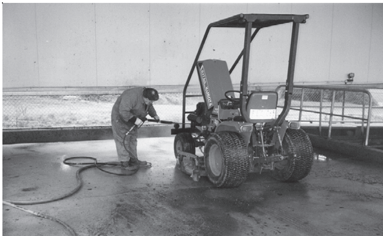
Figure 6.3 A designated wash-down area at the City of Manningham's works depot. A paved, undercover area draining to a sump (City of Manningham).
