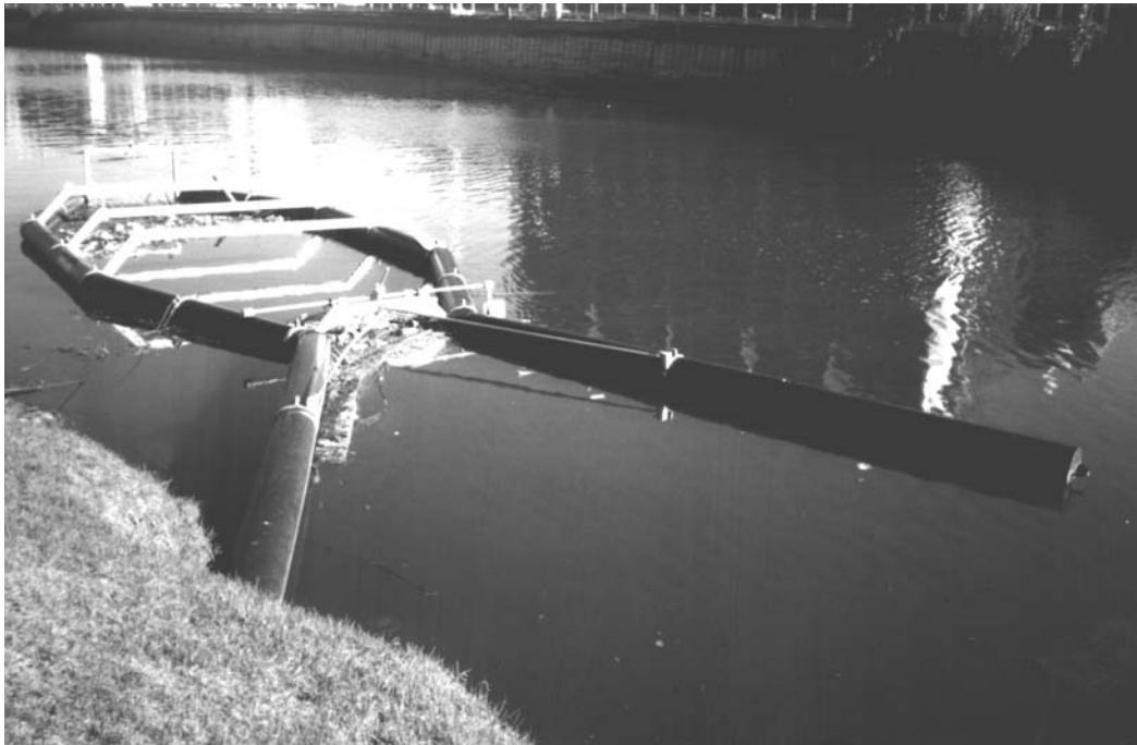
Figure 7.19 Plan view of floating debris trap.
