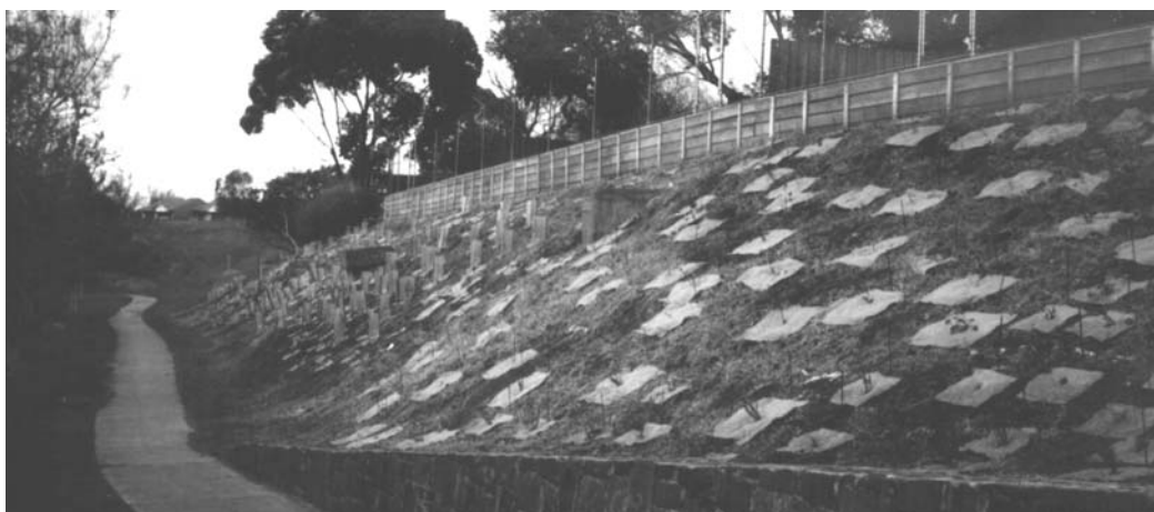
Figure 6.10 Stabilisation and revegetation protect soils from erosion.
