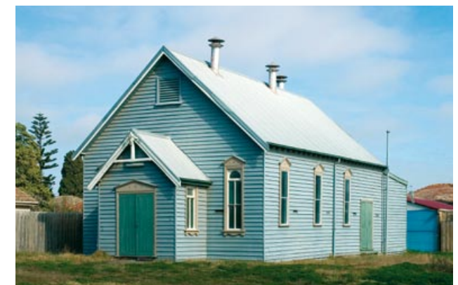
cxxvi Former Methodist Church and Sunday School, 53 Alma Street, Malvern East. [SLHC Reg. No. 9535]
