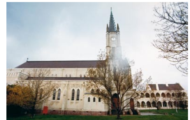
cxxxii Convent of the Good Shepherd, Chadstone, in 1985. Demolished to make way for extensions to the Chadstone Shopping Centre. [SLHC Reg. No. 7734]
