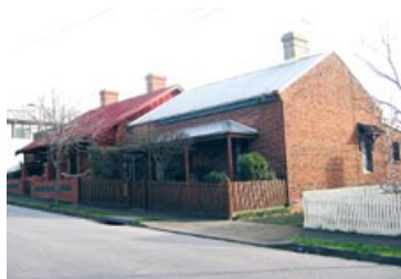
Ixii Tile worker's cottages at 1 and 3 Cawkwell Street, Malvern. [Context 2005]
