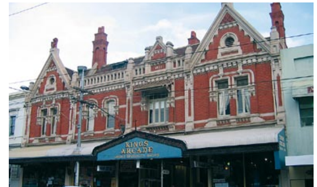
Ixxii Former Armadale Arcade in High Street, Armadale. [Context 2005]
