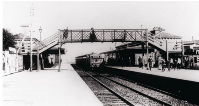
xliv Malvern Railway Station c.1900 [prior to the improvements made when the line was electrified (SLHC Reg. No. 1356) and (right) a view in 1997. (Context 2005)]
