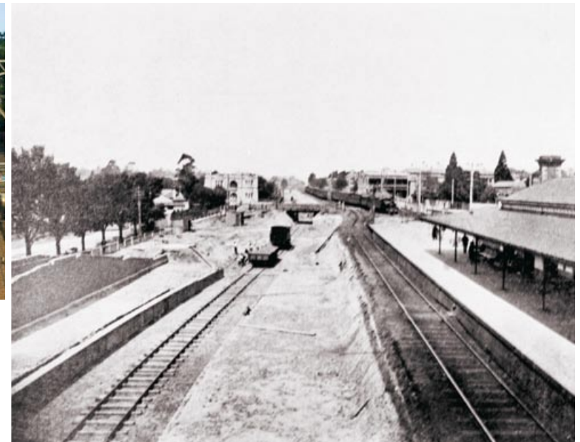
xlv (right) Re-grading of Oakleigh railway associated with electrification at Hawksburn Station c.1915 looking east toward Williams Road. The new line is the lower one on left (SLHC Reg. No. 8894) and (above) a similar view today, also looking east. (Context 2005)
