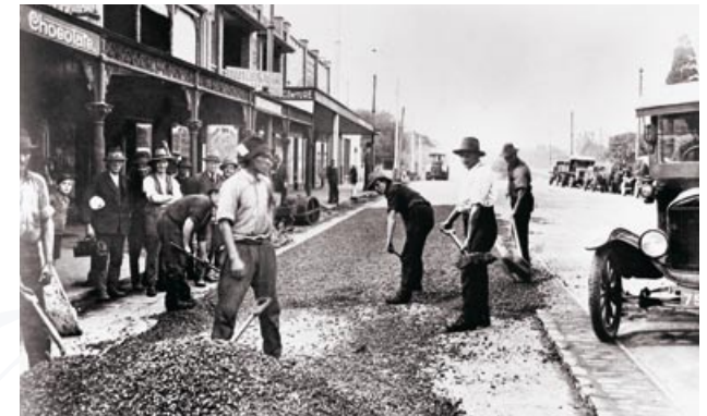
xliii Roadworks in Dandenong Road, east of Chapel Street, c.1910. [SLHC Reg. No. 8646]
