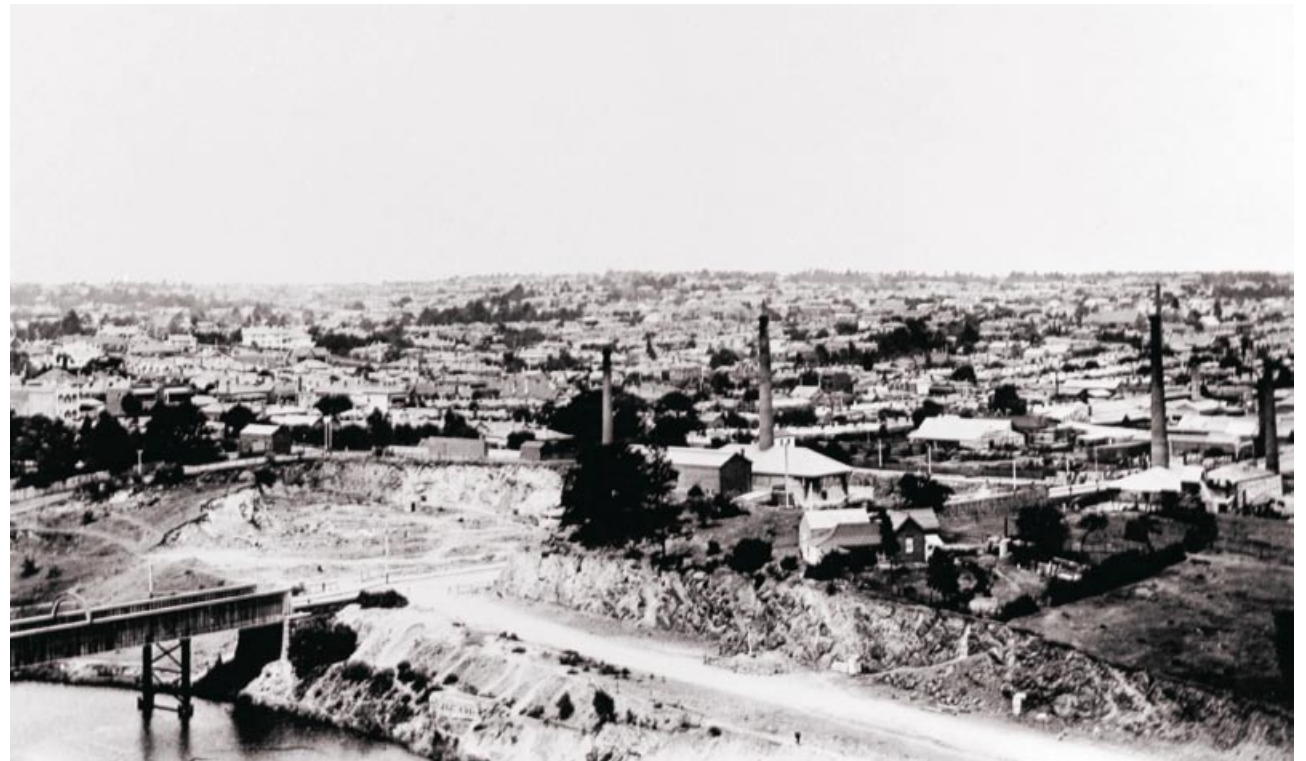
xii View c.1915 looking south-east toward South Yarra showing the quarry that removed Forrest Hill on the east side of Chapel Street. The image also shows the first stage of construction of Alexandra Avenue. The chimneys show the brickworks associated with the quarry. [SLHC Reg. No. 7101]
