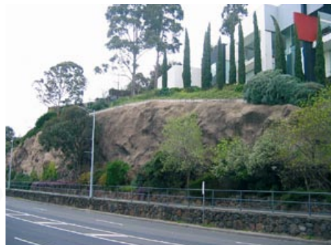
xiv (right) View c.1931 showing excavations to allow construction of Alexandra Avenue east of Chapel Street [SLHC Reg. No. 6151] and (above) c.2005 the cutting as it appears today. [Context 2005]
