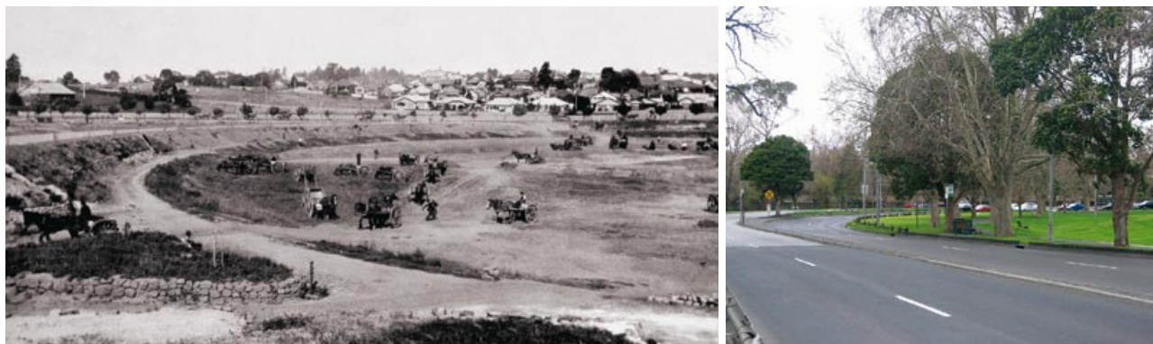
xvi Regrading works at Como Park c.1932. This view looking south-east shows the sweeping curve of the new levee bank road connecting Williams Road with Alexandra Avenue [SLHC Reg. No. 6144.11] and (right) a similar view today. [Context 2005]
