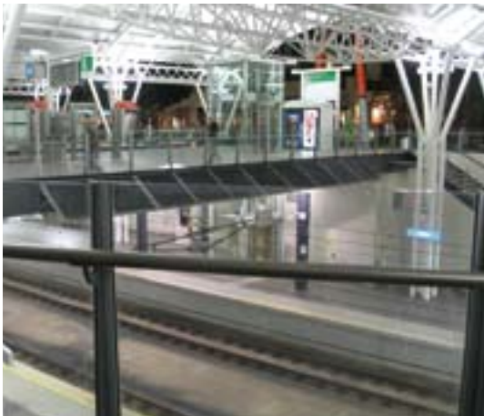
Figure 4: Subiaco Railway Station - WA
