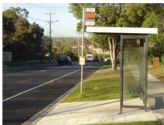
Figure 25: Continuous accessible pedestrian path
