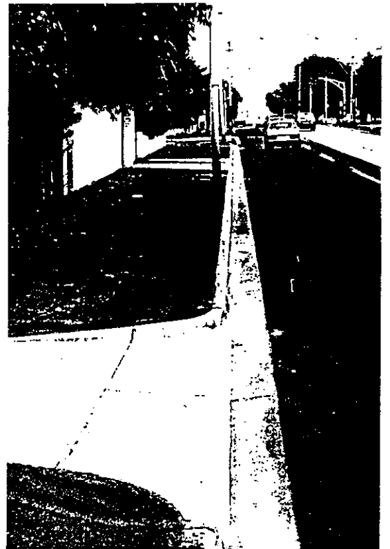
HIGH STREET SHOWING CONCRETE KERB & CHANNEL WITH ASPHALT PATH.
