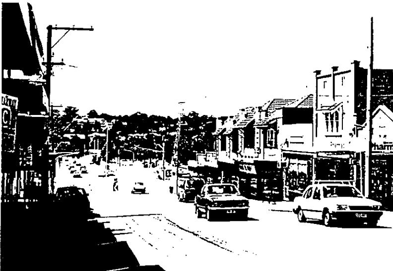
HIGH STREET GLEN IRIS SHOWING NEW ROADWORKS.
