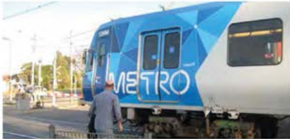
Railway crossing - uninviting pedestrian movement
