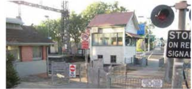
Railway crossing and signal box - potential heritage value requiring retention (No 3A)
