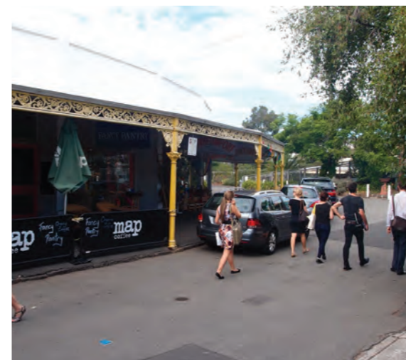
Single storey period built form adjacent to the railway line
