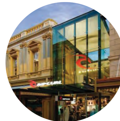
new infill building should reflect the existing parapet line
