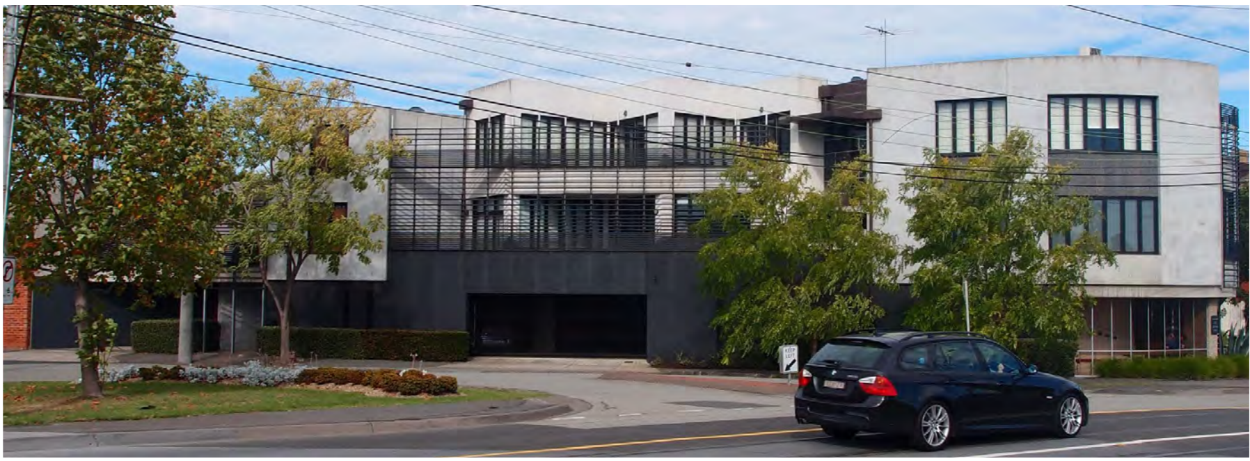
Existing residential development within Study Area
