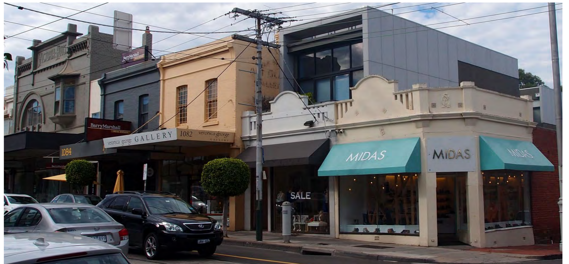
Existing mixed use development within Study Area
