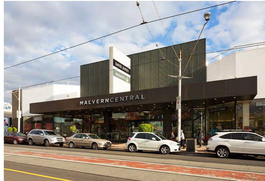
The implementation of a 40km/h limit through the centre would increase safety for pedestrians and cyclists
