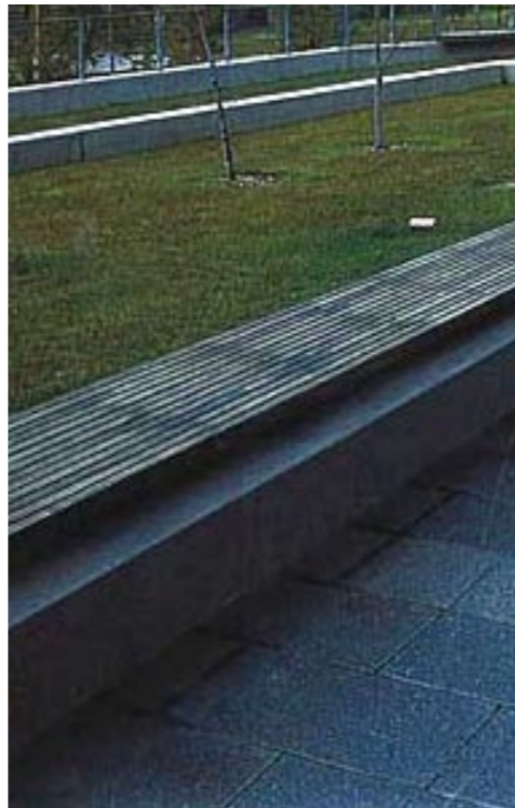
Timber battens on precast concrete base
