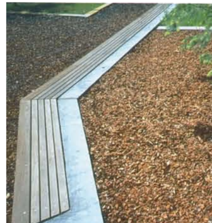
Insitu concrete steel wall with timber
