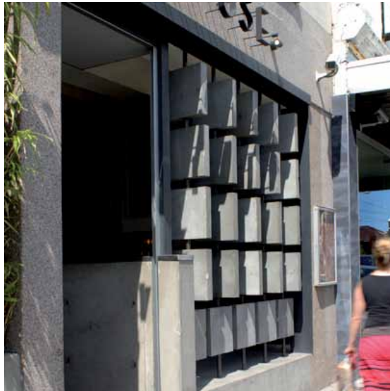
doors and windows should not allow patrons to spill out onto adjoining public spaces
