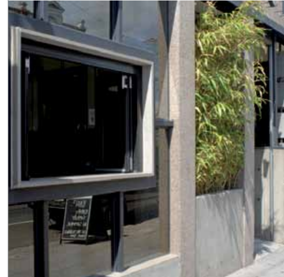
maximise opportunities for passive surveillance of public spaces through the use of design options including windows and balconies
