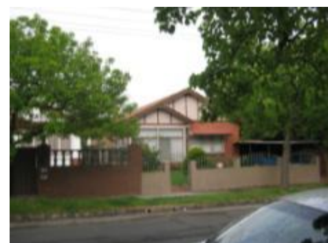
Figure 3.3: Dwelling on south side of John Street
