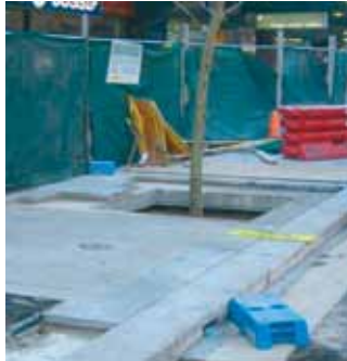
Construction of a planter tree
