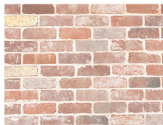
BR 4 Red Brick recycled from site building with lime wash
