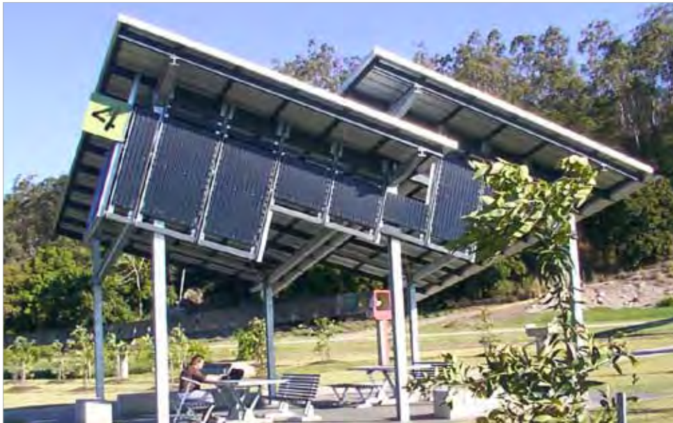
Environmentally Conscious Public Realm Park structures can be used for solar generated electricity Park pavilion at Rodes Park, Brisbane. Designed by Brisbane City Council (Source: ASPECT Studios)
