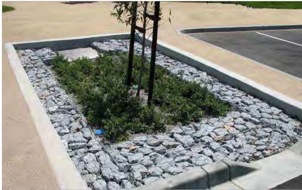
Water Sensitive Urban Design Tree pit Docklands streetscape, Melbourne (Source: ASPECT Studios)
