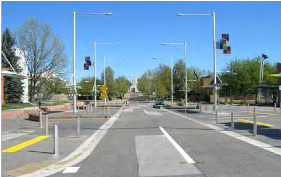
Shared Surfaces Shared surfaces provide the potential to increase pedestrian and cyclist movement in the public realm Street in Canberra where the removal of kerb allows easier pedestrian movement in a safer road environment. Designed by EDAW (Source: ASPECT Studios)
