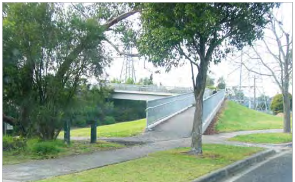
Pedestrian Links Pedestrian Links over Monash Freeway, Glen Iris (Source: ASPECT Studios)
