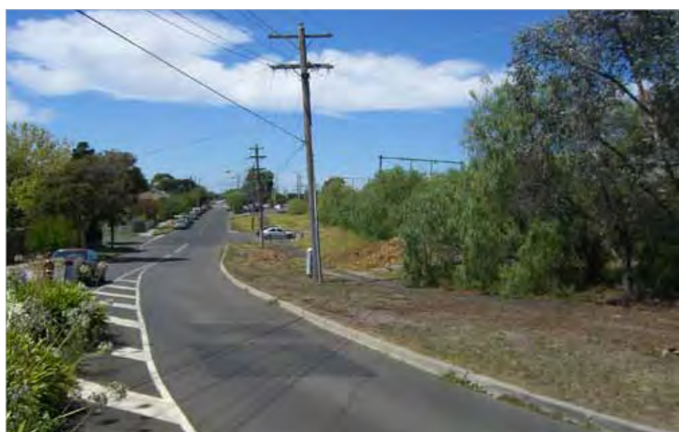
Public Space Challenges Path adjacent to Glen Waverley line (Source: ASPECT Studios)
