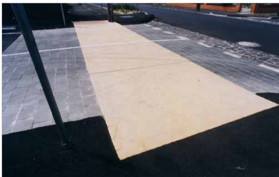
Shared Pathways Raised pedestrian and cyclist shared pathway over local road Albion Street, Coburg (Source: ASPECT Studios)
