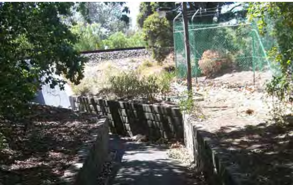
York Road Underpass (typical link under railway and freeway). Source: ASPECT Studios
