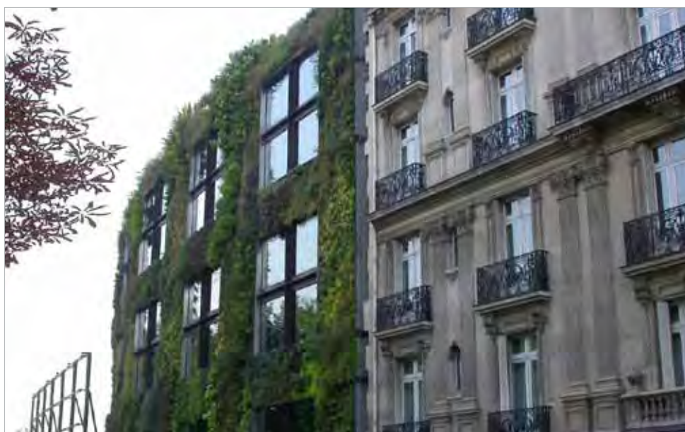
The Private Realm The private realm contributes significantly to the amenity, function and health of the public realm Green walls on buildings provide increased thermal performance for the building and a great 'green' addition to the streetscape Patrick Blanc Green Wall, Paris (Source: ASPECT Studios)
