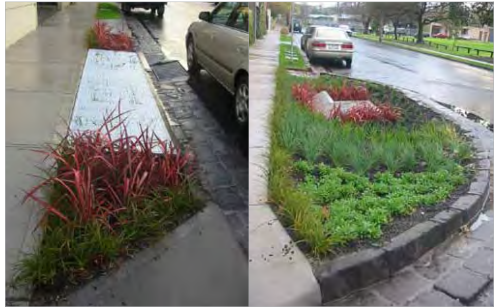
Water Sensitive Urban Design street gardens in Stonnington (Source: City of Stonnington).
